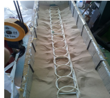
(c) Installation of pipe
